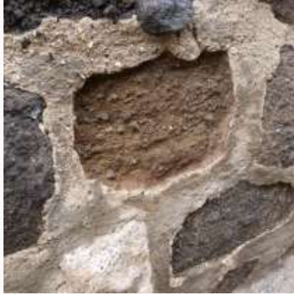
Joints ciment. Gros plan.
